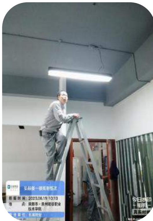
弘毅楼一楼照明整改
